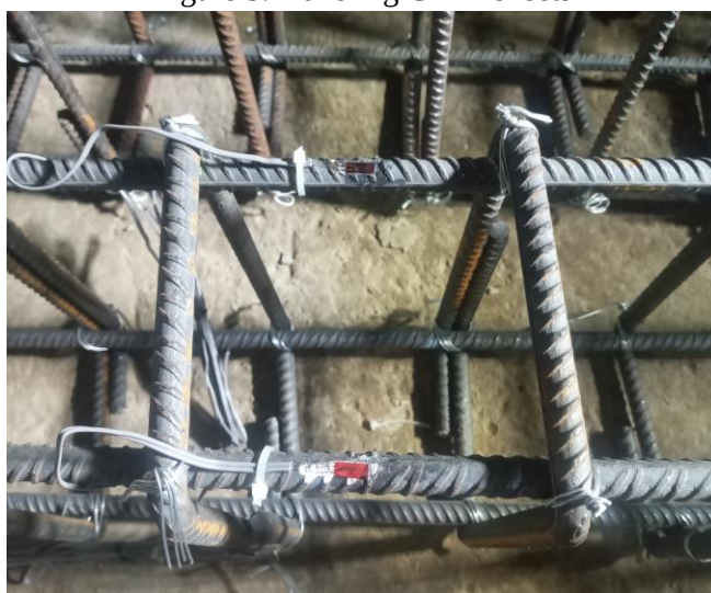
Figure 4. Strain gauges installed on the tensile reinforcement
