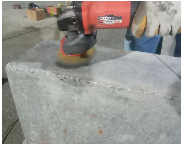
Figure 2. Beam soffit preparation before CFRP sheets are installed
