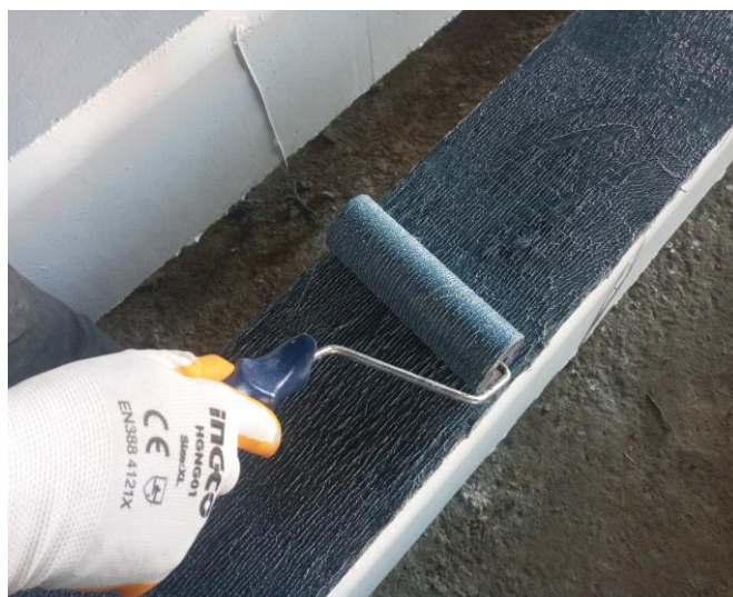
Figure 3. Adhering CFRP sheets
