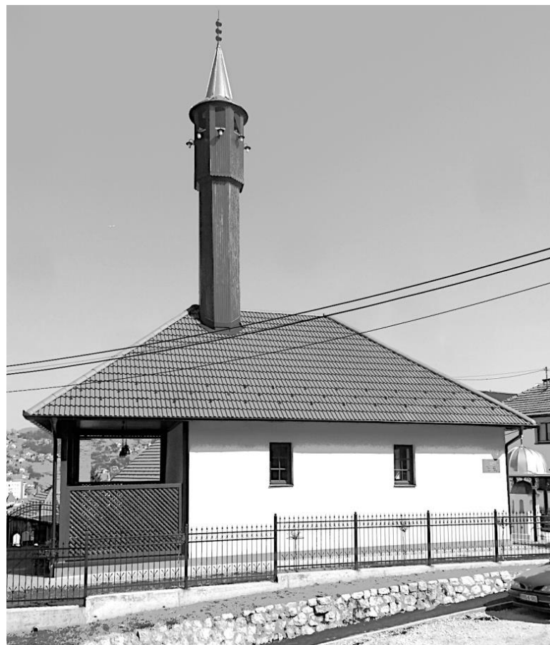
Figure 5. Osman Ćehaja Mosque after the renovation (Photo by the author)
