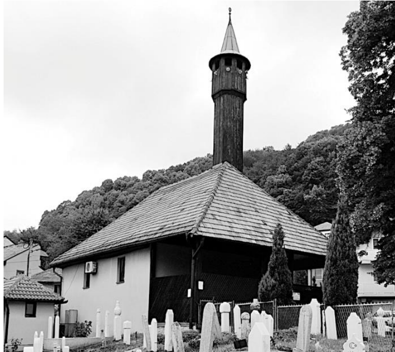
Figure 4. Osman Ćehaja Mosque in Tuzla before the renovation (Photo by the author)
