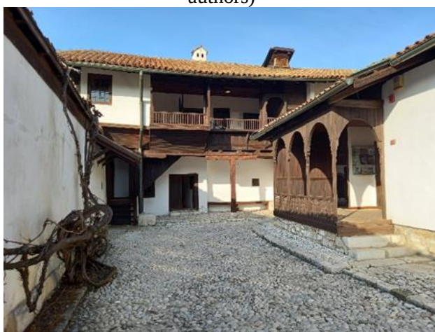
Figure 9. Selamluk with courtyard (Source: authors)
