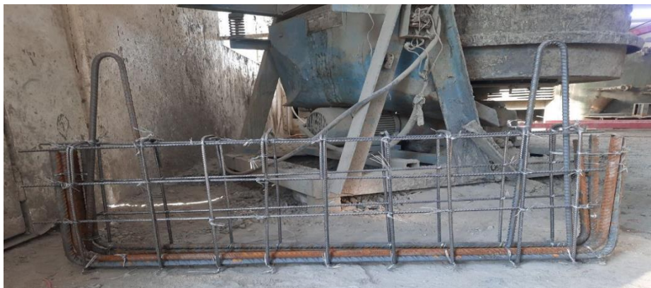
Figure 3. Steel reinforcement cage used in deep beams
