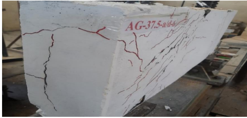
Figure 7. Crack pattern for beam (AG-37.5-a/d-6)
