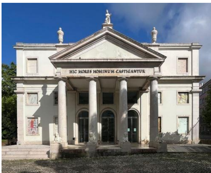
Figure 7. image of the south façade after restoration
