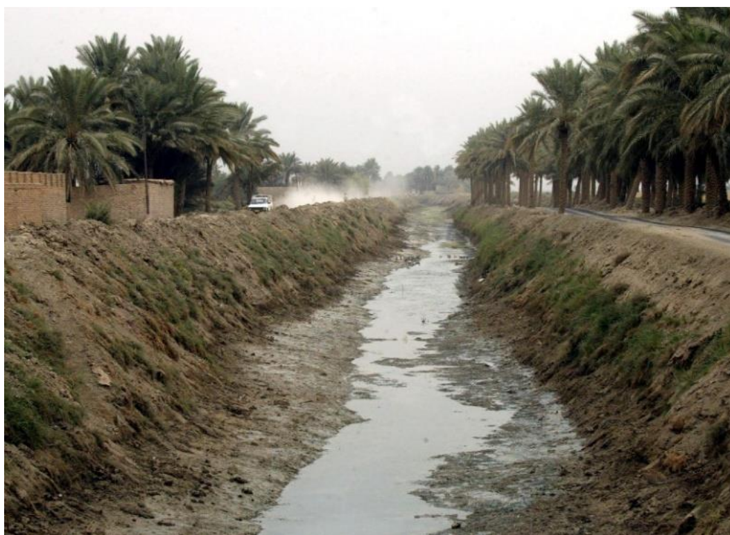
Figure 1. Inlining canal in Mishkhab area
