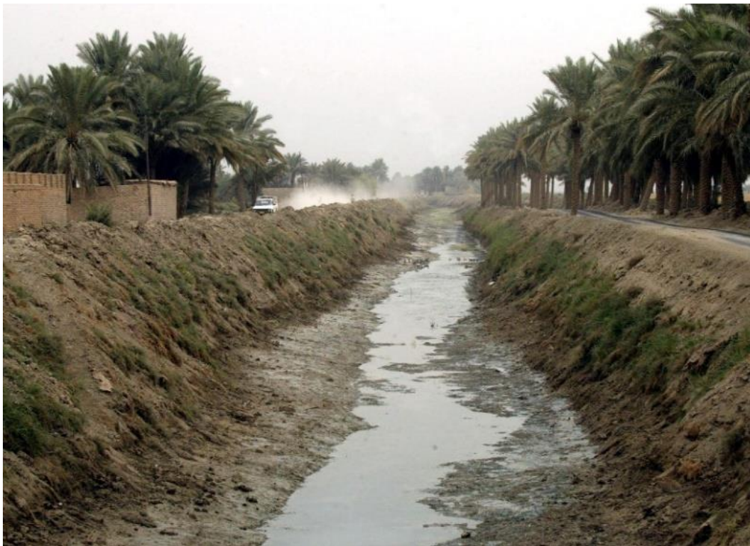
Figure 1. Inlining canal in Mishkhab area
