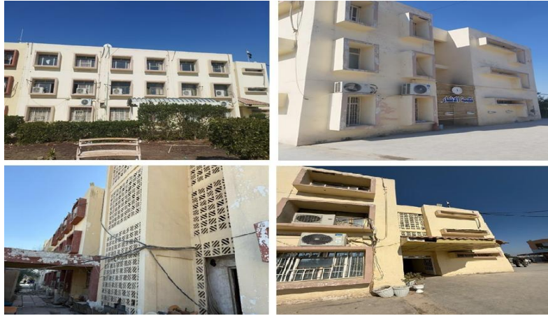
Figure 1. Faculty of Arts Building (B), Al-Qadisiyah University, Al-Diwaniyah, Iraq: existing condition (on-site photographs showing uninsulated façades, split-unit AC condensers, and the decorative concrete screen panels)
