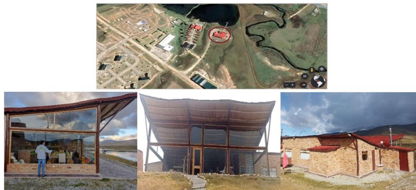
Figure 1. Aerial, front, side and rear view of rural housing in the case study
